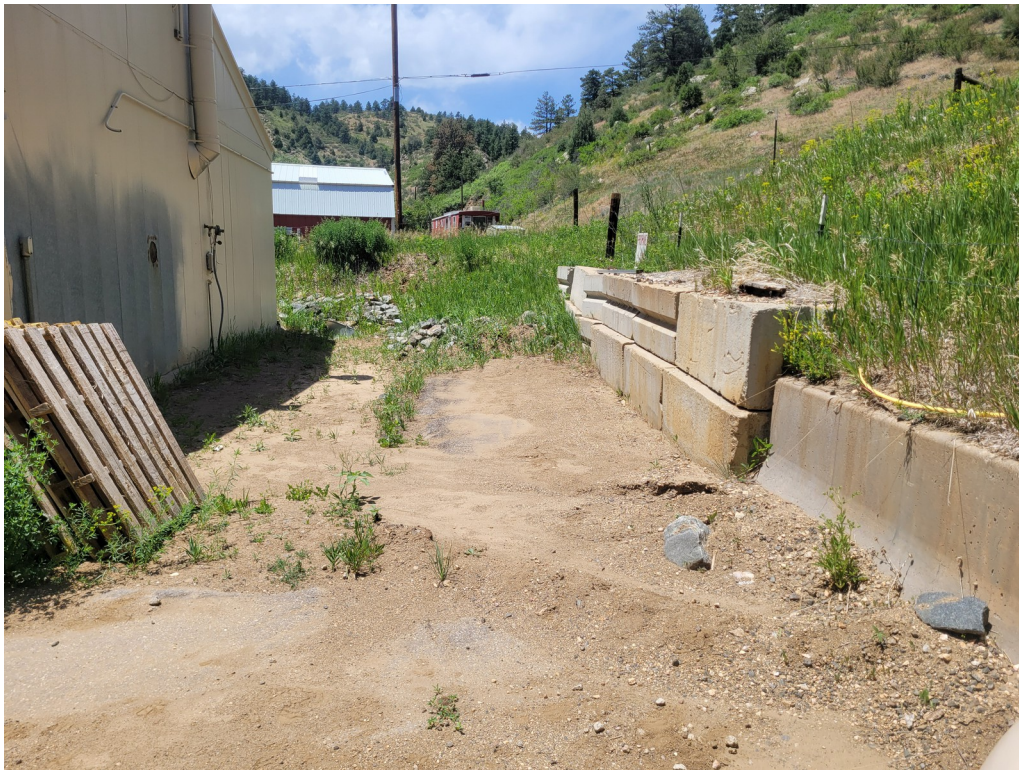
Image 4 – Sediment deposition behind the station
