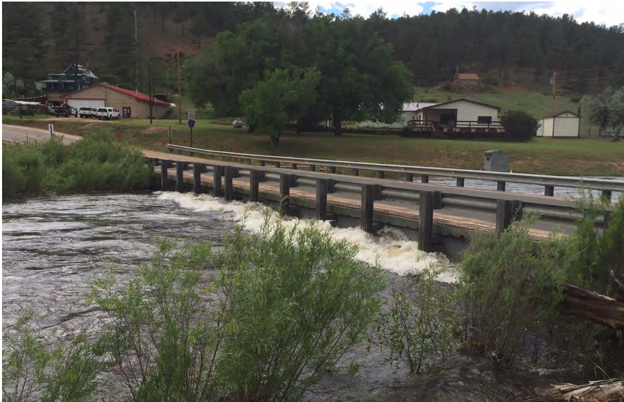
Figure 4-29 South Platte River at Trumbull Bridge Hwy 67 June 17, 2015
